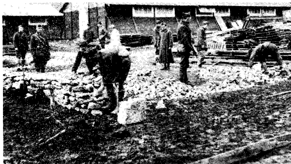
Engineers lay the foundation for a field hospital building at Ménil-la-Tour (Meurthe-et-Moselle), France.
