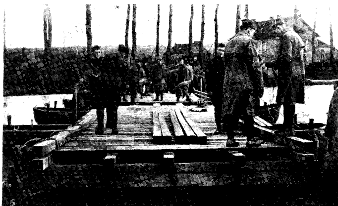
Engineer troops build a ponton bridge in France
