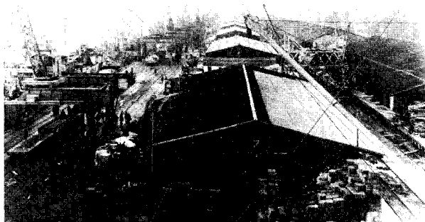
The derricks at this American-built dock at Bassens could lift cargo from ship holds and place it directly in waiting railroad cars.
