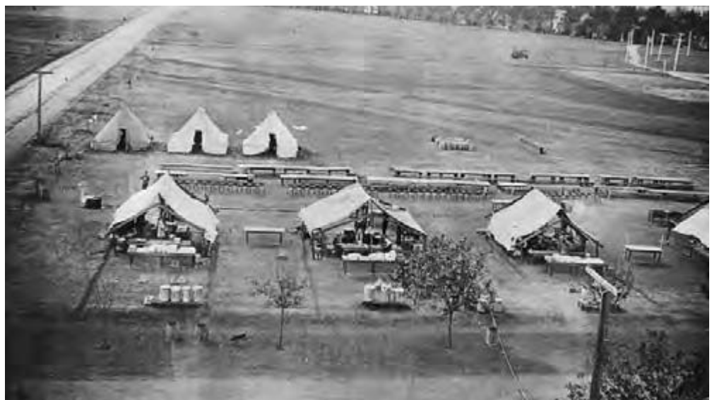
Stanford received $25,000 for leasing its property for Camp Fremont. The government paid to construct the camp, working with firms recommended by local civilian advisers.
